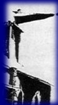
This is the Steeple coming down during the remodeling of the Church in 1936.
